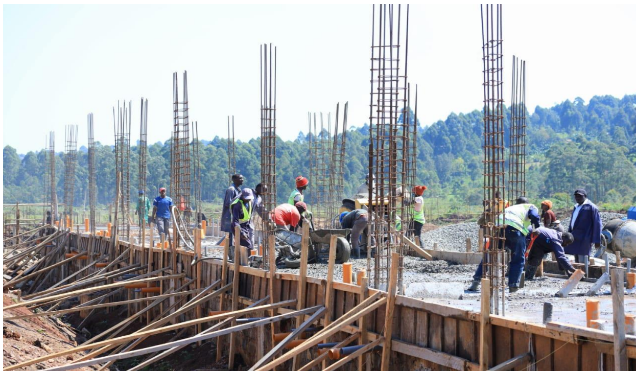
Construction of 8 units at Sironga industrial park
