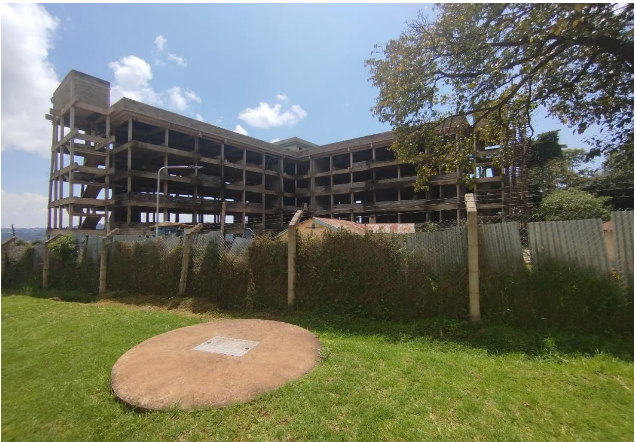
Ongoing construction of county headquarters
